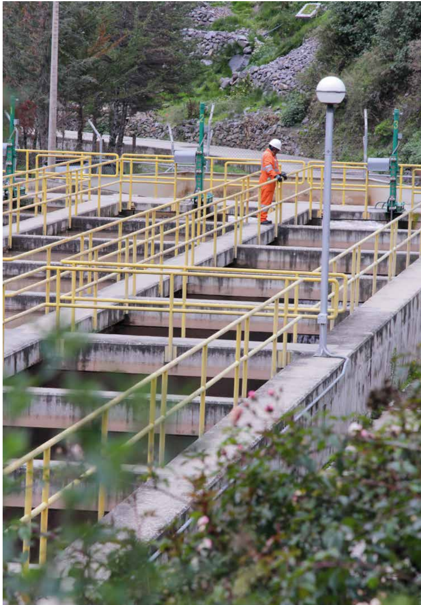
Desander - Huanchor Hydroelectric Plant
