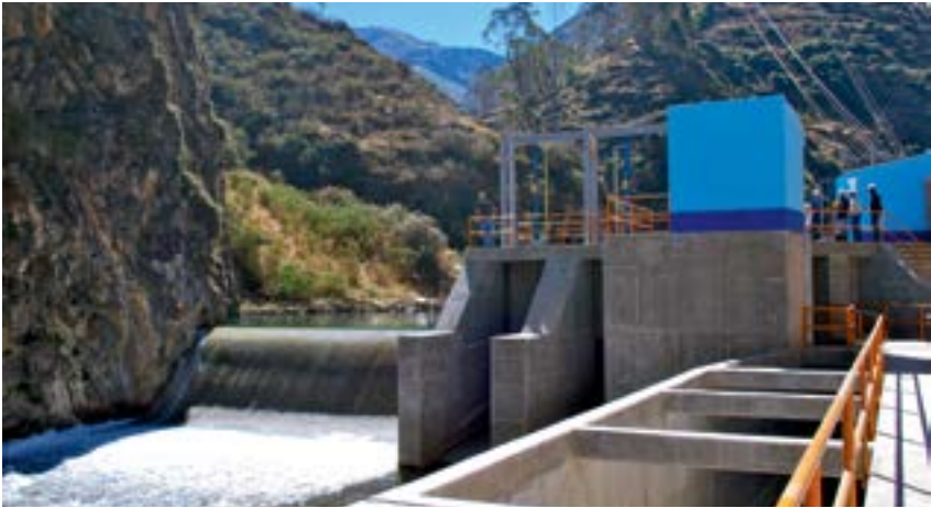
Water intake for Baños V Hydroelectric Power Plant.
