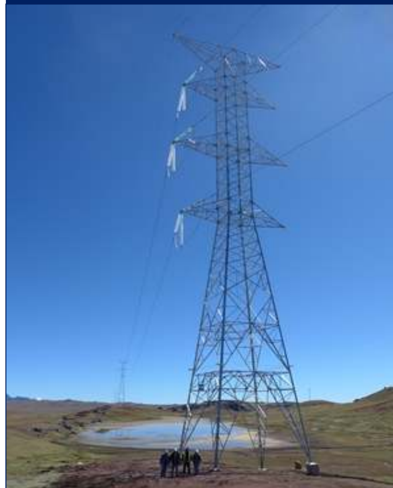
Paragsha II – Francoise Transmission Line 45 km – 118 towers
